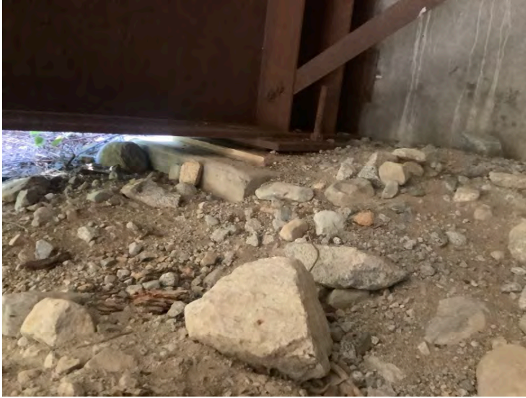
Right Bank Abutment when facing downstream
