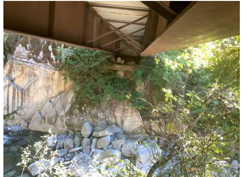
Left Bank Abutment when facing downstream
